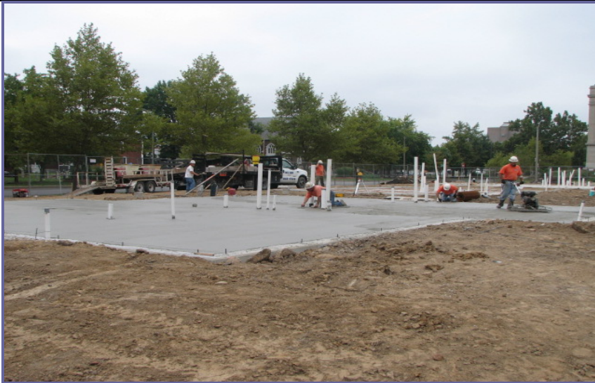
Laying foundation for Kingsway Townhomes at 2301-2323 N. Kingshighway
